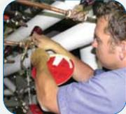
We adjust the water networks (pumps, water towers, exchangers, chillers, coils, valves...) so they perform according to prescribed requirements. We use portable ultrasonic flow meters or hydronic pressure gauges to measure the fluids' flow. The sophisticated instruments used by our technicians are calibrated on a periodical basis. The certificate of calibration can be provided upon request.
